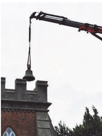
Saint Peter's bell being lifted from its place in the tower this month and onto a waiting truck in preparation for earthquake strengthening of the upper section of the tower.
