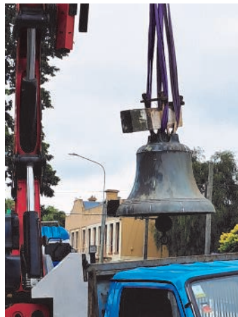
Saint Peter's bell being lifted from its place in the tower this month and onto a waiting truck in preparation for earthquake strengthening of the upper section of the tower.
