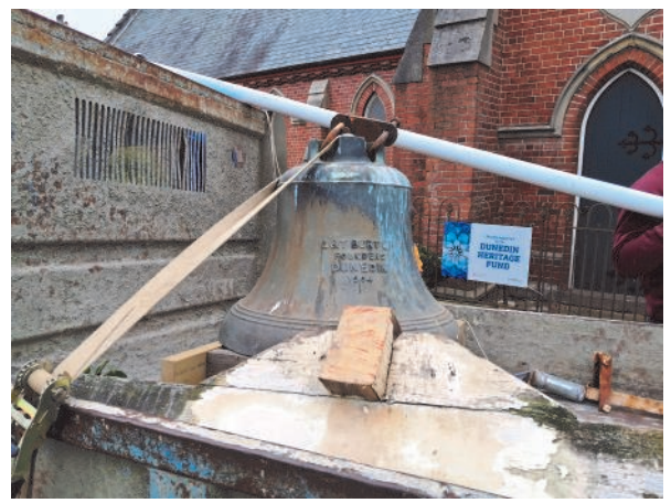
Saint Peter's bell being lifted from its place in the tower this month and onto a waiting truck in preparation for earthquake strengthening of the upper section of the tower.
